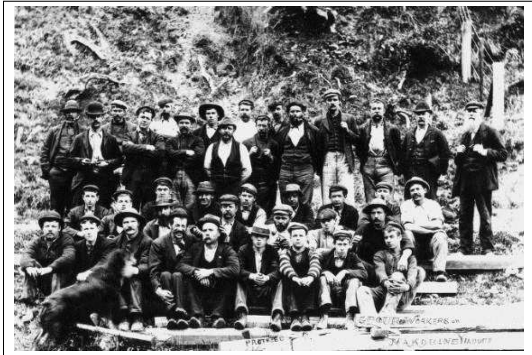
Figure 2: Makohine Viaduct Workers, between 1898-1902. Cameron, R A: Photographs of Ohingaiti, ATL, ID:1/2-094227-F.
