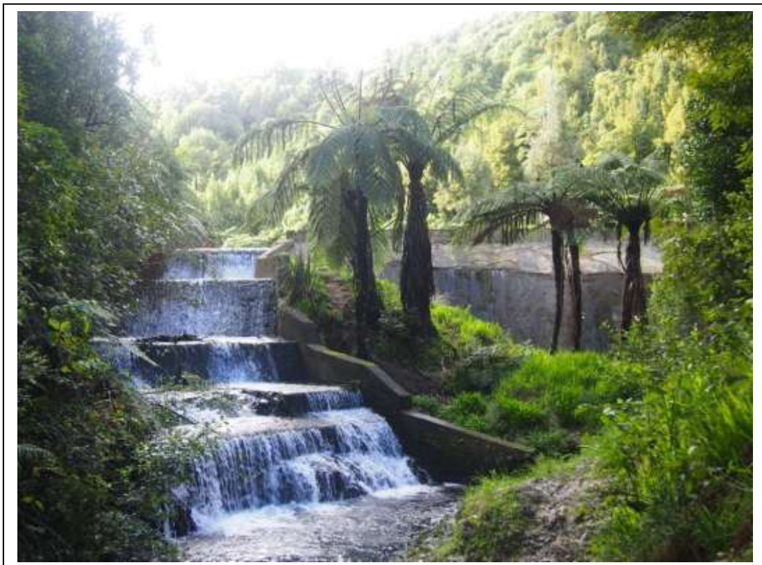
Korokoro Dam, Belmont Regional Park, Wellington. Karen Astwood (IPENZ), 28 August 2013.
