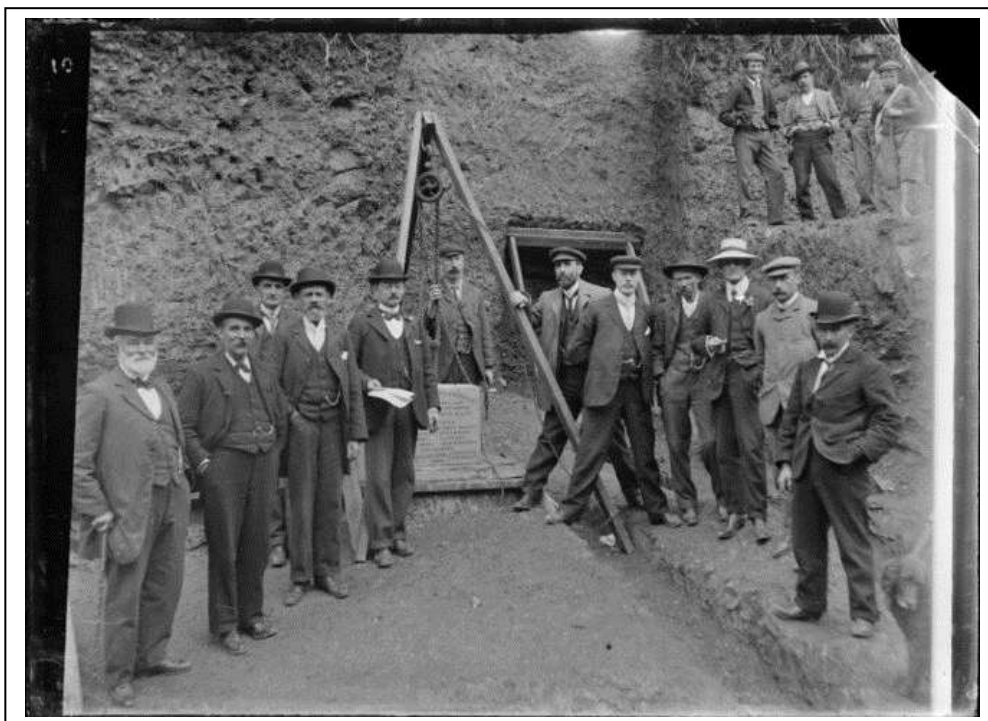
Figure 3: Officials at the laying of the Foundation Stone for the Petone Waterworks, 25 April 1903. Godber, Albert Percy, 1875-1949: Collection of albums, prints and negatives. Ref: APG-0071-1/2-G. Alexander Turnbull Library, Wellington, New Zealand. http://natlib.govt.nz/records/22735327 . Permission of the Alexander Turnbull Library, Wellington, New Zealand, must be obtained before any re-use of this image. Jickell is standing behind the men on the left of this image.
