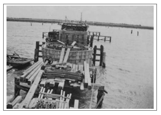
**Figure 5:** Kopu Bridge under construction, *circa* 1928. Photographer: John Isdale. Image courtesy of Thames School of Mines, Thames. The swing span's concrete pier is at the centre of the image.
