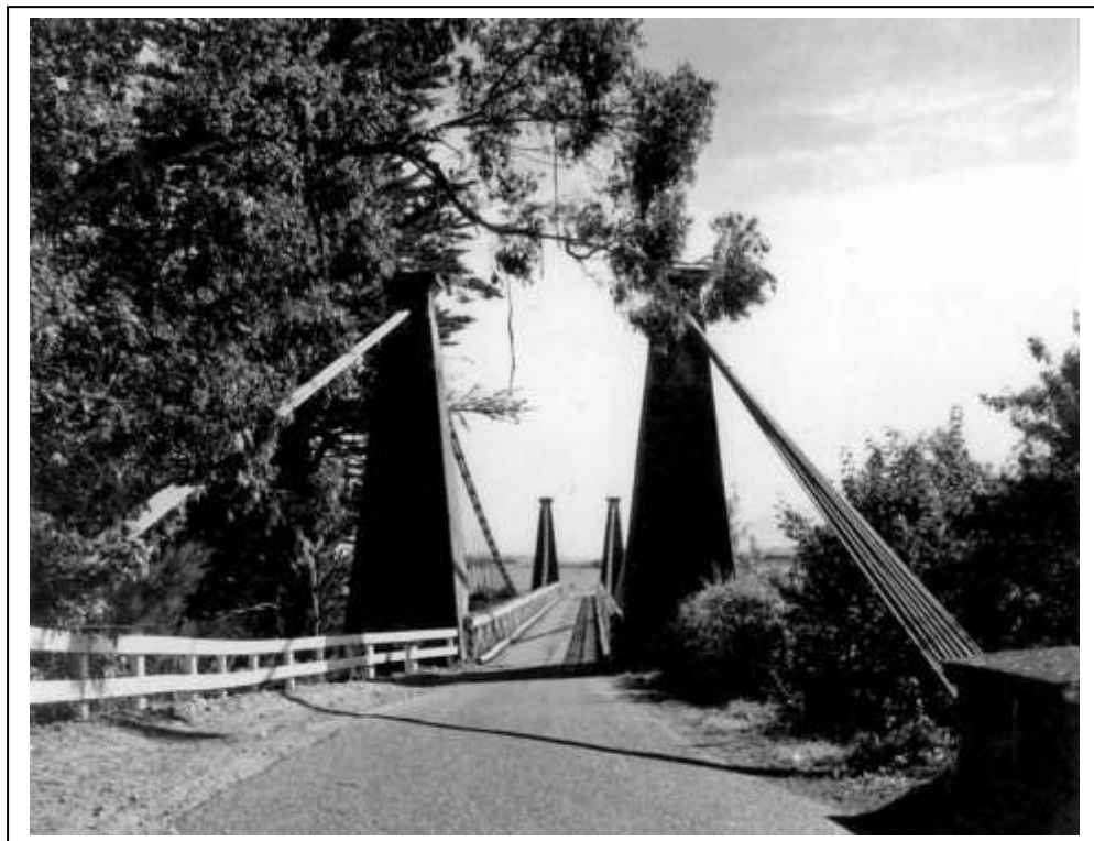
Figure 5: Clifden Suspension Bridge, date unknown. Geoffrey Thornton Photograph Collection, IPENZ
