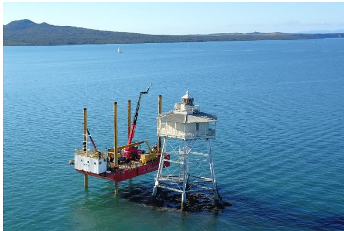
Figure 3: Jack Up Barge (JUB)
