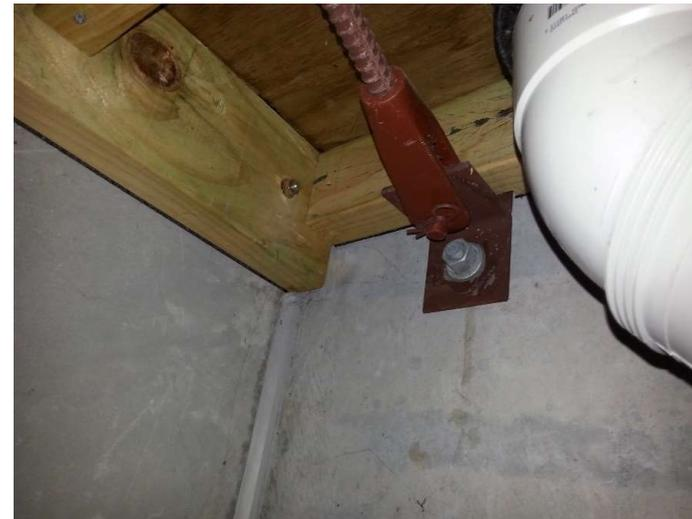
**This connection cannot transfer the loads required & is not a recommended detail**
