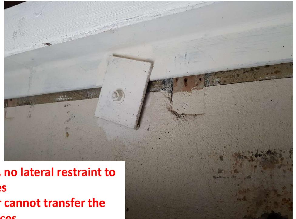
**Eccentric connection to panels, no lateral restraint to PFC flanges**
