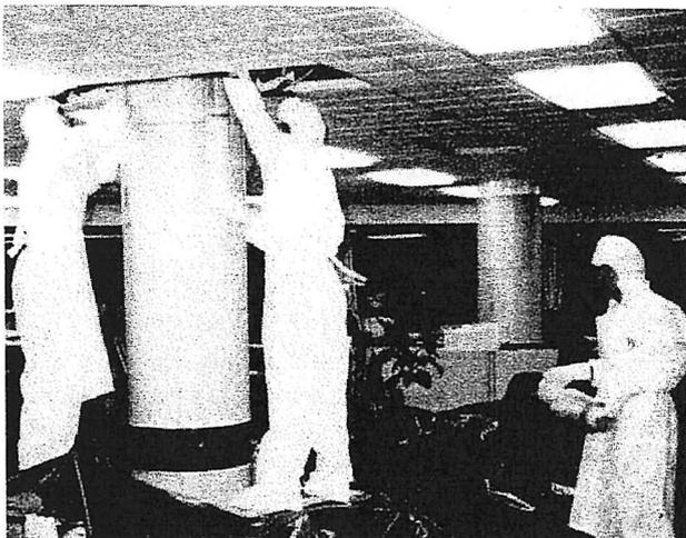
**Fig 8: Application of pre-saturated ACM to interior column of a multi-storey building**
