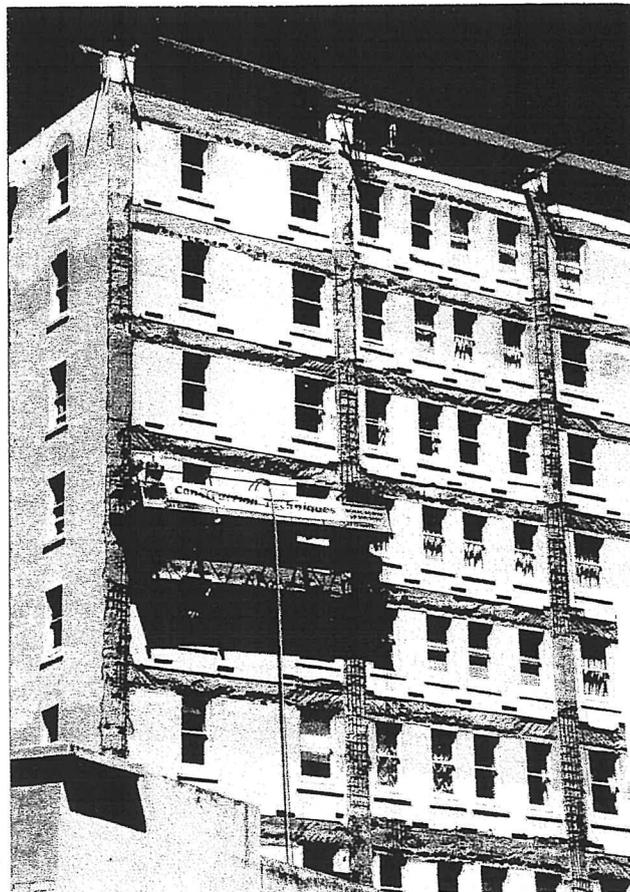
*Fig 4: Westminster Court Apartment – state of the concrete and reinforcement prior to the repair and application of a CP system – 1989*
