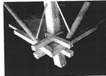
Figure 7 The corner clamp - anchors prop to building
