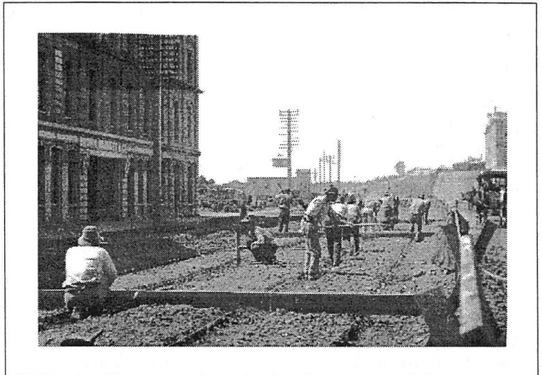
A grading gang at work in Customs Street East. Trenches are being excavated for the longitudinal concrete stringers supporting the rails. This form of permanent-way construction was not successful and was eventually replaced by transverse timber sleepers.
