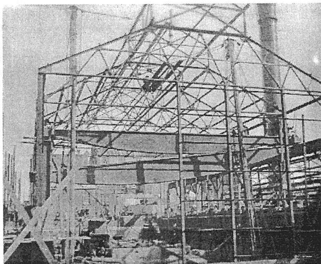
The power-house was erected and completely fitted out with the generating plant in four months. A simple derrick was used to lift all the building components, including the 20-ton gantry girders as shown here.
