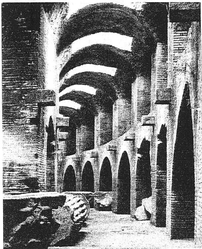
*Fig 3: Amphitheatre at Pozzuoli shows both the engineers' highly developed use of arches in their design and the strength of their concrete standing firm after 2000 years even if some of the brick facing has fallen*
