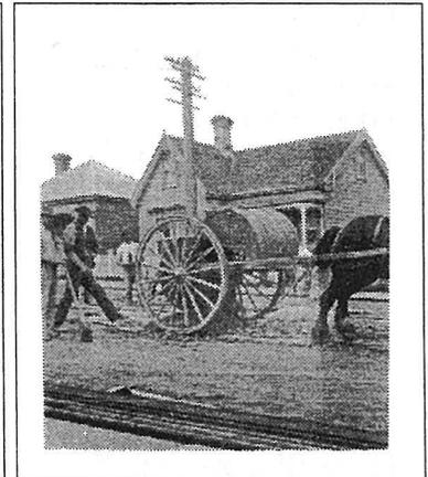
Left: Filling the concrete mixer. Right: After taking the horse for a walk, the concrete is dumped to form the longitudinal stringers
