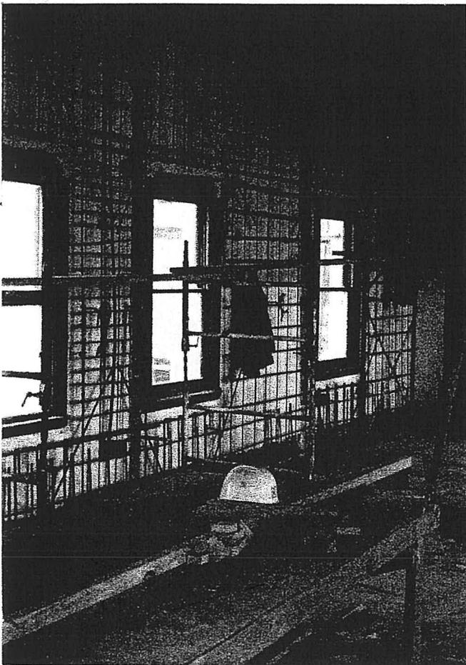
*Fig 5: Typical preparation of a masonry walled building prior to the construction of new reinforced concrete walls to which the masonry walls are attached. Wall construction is by sprayed concrete – Baradene College, Auckland*
