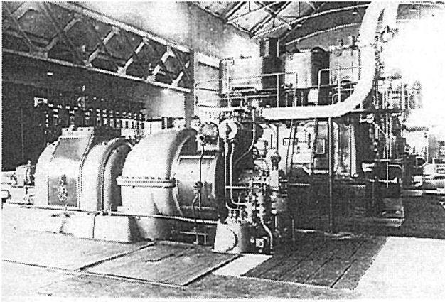
**Figure 2 Machine Room with Bellis & Morcom Engines and BTH Turbo alternator**
