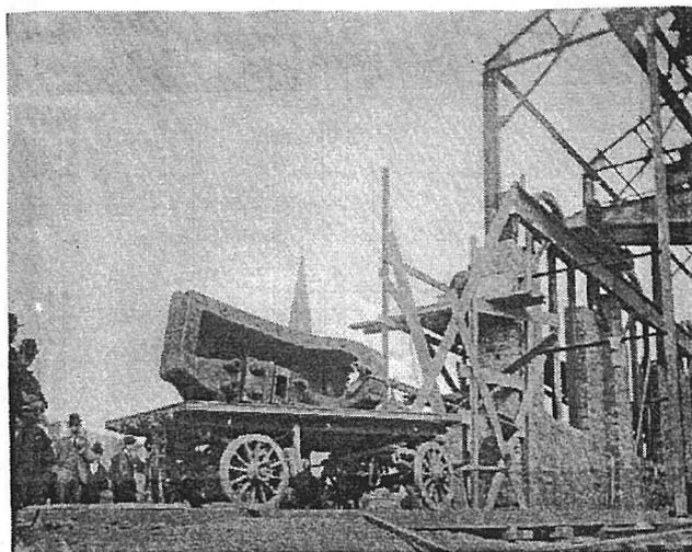
An engine frame is delivered to the power-house by J J Craig. It will be lifted into place with the newly installed gantry.
