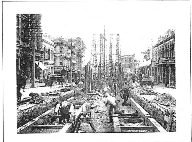
Not all of the original work was a success. Major foundation problems in Queen Street required extensive piling in 1906 – shown here. Failure of concrete packing beneath the rails entailed more major remedial works in 1913.
