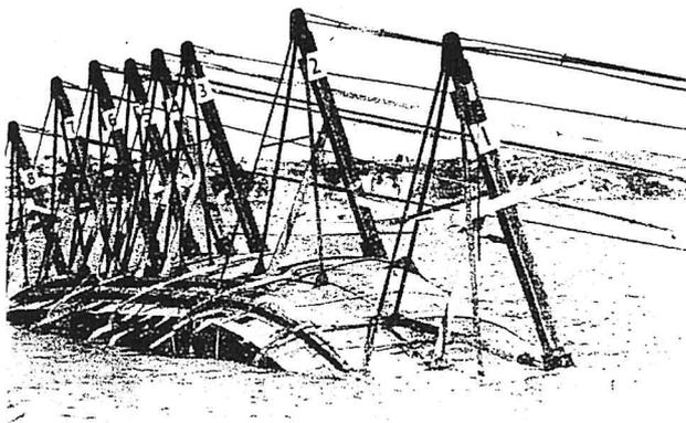
Fig. 1: Eight frames 20 ft high in position on the hull (October 1, 1957); pull of 320 tons causing initial rotation. - "N.Z. Herald" photo
