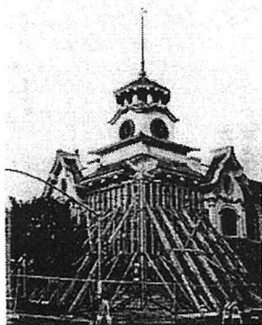
Figure 4 Propping an earthquake damaged building copyright permission still in progress
