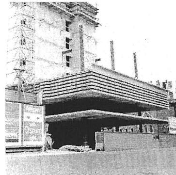
Figure 3 Lift slab construction in-progress
