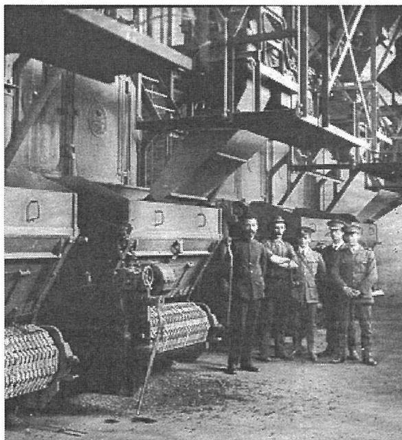
**Figure 5 Babcock and Wilcox Boilers with Chain Grate Stokers at Kingston Powerhouse**
