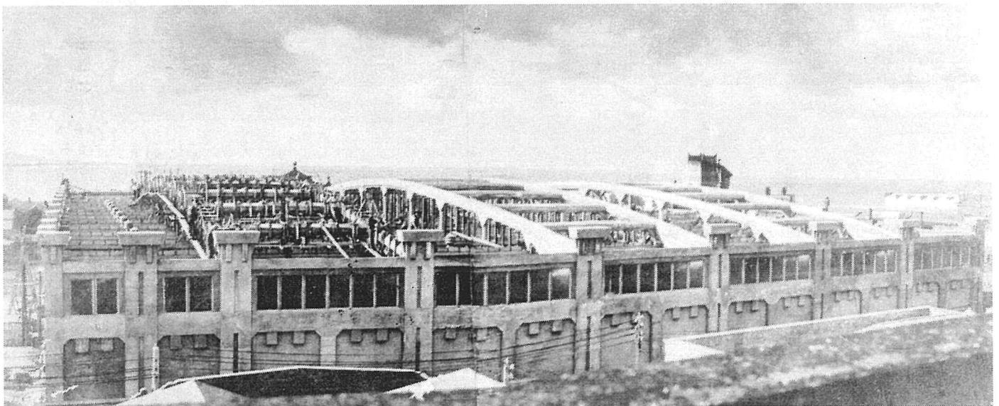
Figure 2 - Roof of Wool store under construction in 1910
