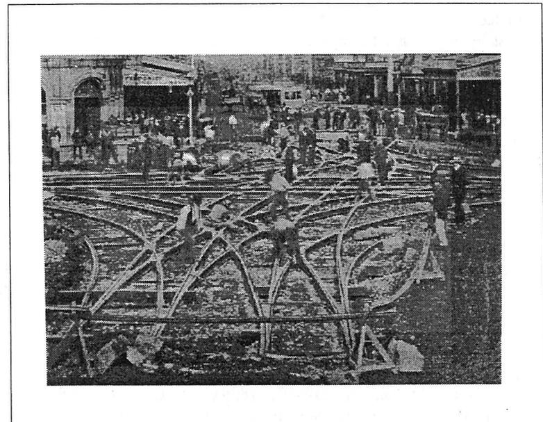
Laying out the many components of the "grand union" at the junction of Queen and Customs Streets. Trams approaching in any direction could turn left, right or continue straight on. Grand unions were rare even in large tramway systems. Another was installed at Queen and Wellesley Streets in 1916 with the construction of the upper Queen Street section.
