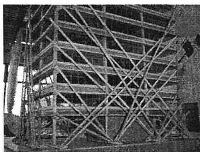
Figure 5 Propping against the face
