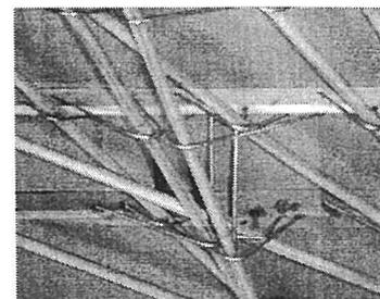
Figure 8 The bow tie - prevents buckling
