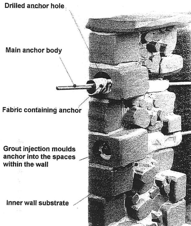
*Fig 10: Functioning of standard Cintec anchor within a masonry wall.*
