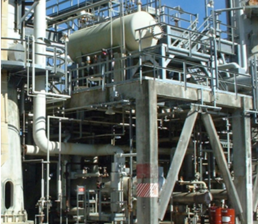
Figure 3: Vessel support structure.
