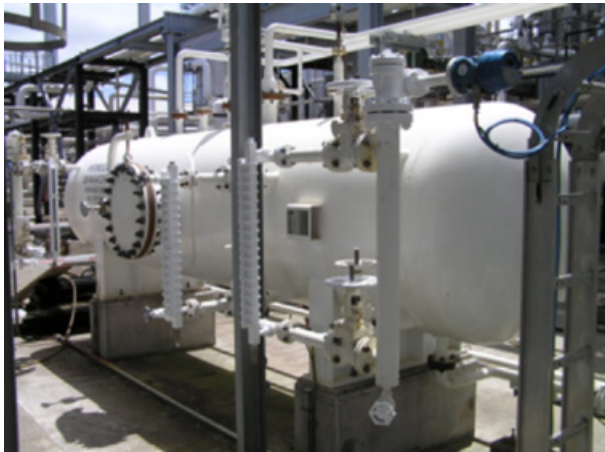
Figure 1. Horizontal pressure vessel on short pedestals
