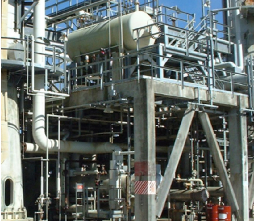
Figure 3: Vessel support structure.
