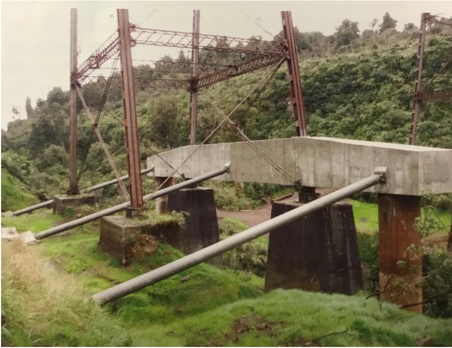
Showing the new piles and crossbeam. Photo: "Makatote Viaduct – Underpinning Pier 7," Concrete , Vol 51: 4 (December 2007): 1.
