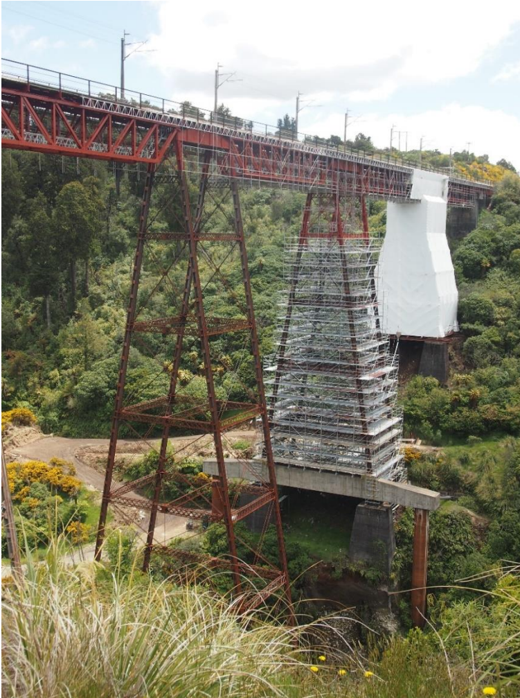
Showing the scaffolding in place during the 2014-2016 restoration work. The 1959 coat of red lead primer was removed, and the piers covered during this process to prevent lead escaping into the environment. Photo: K. Astwood, 26 November 2015.
