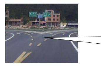
Where is the roundabout? There is no traffic control and you can have head-on collisions either way you turn. The following photos identify other safety issues found on the same project
