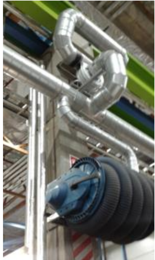
Figure 2: LEV for a diesel exhaust
