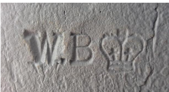
[Figure 22 and 17] Two variations of a works stamp on a joint plate and on a tie-rod. Photo by the author.
