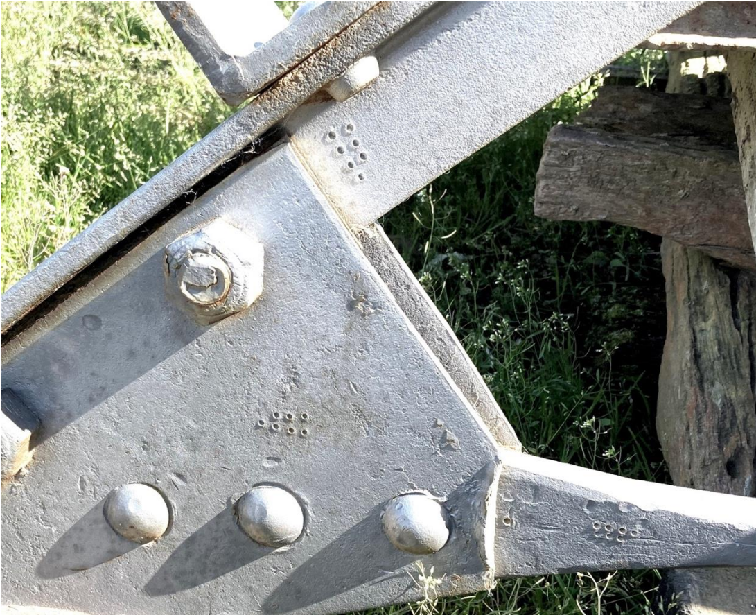
[Figure 19] Joint 7 with dot markings visible on each member. Note the This is the opposite end of the truss that has Joint 8. Photo by the author.
