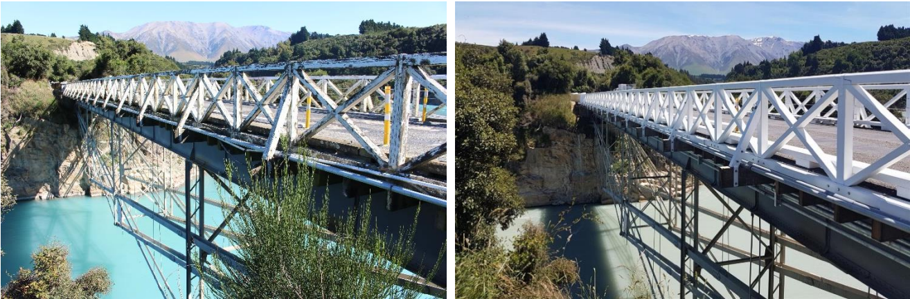
Left: [Figure 17] The damaged balustrade prior to repair. Right: [Figure 18] The repaired balustrade.
