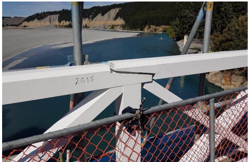
Right: [Figure 26] Installation of the new balustrade with interlocking design.
