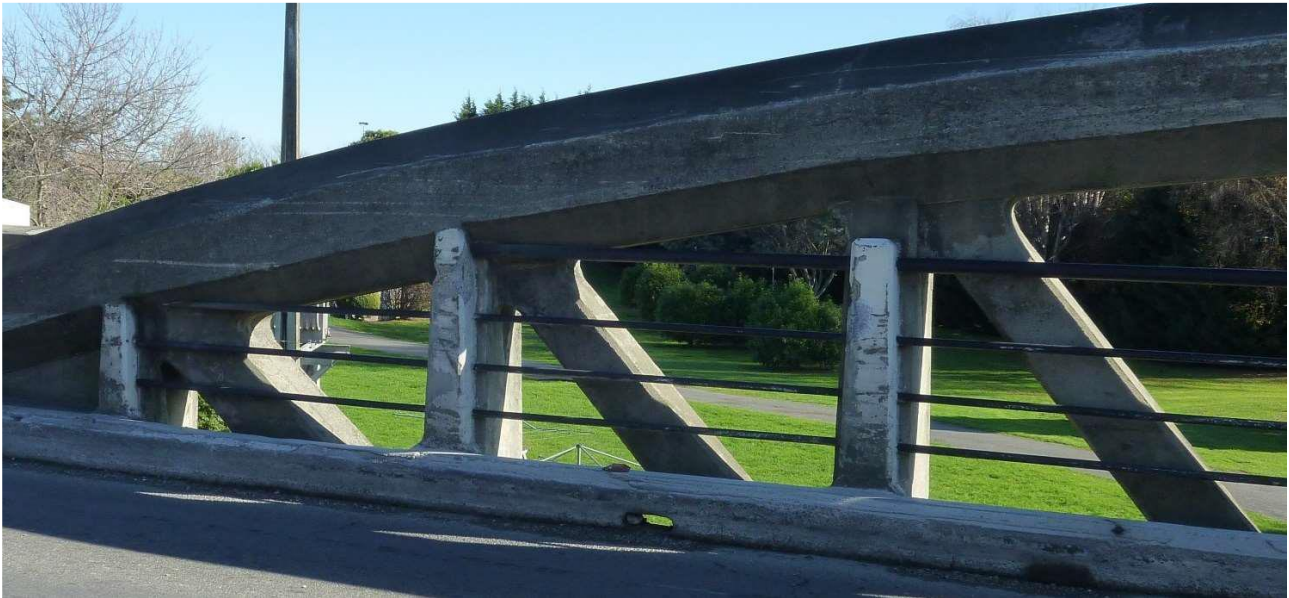
[Figure 40] Mechanical damage to the Opawa Bridge resulting from vehicle scraping and impact.
