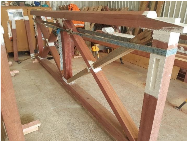
Left: [Figure 23] Reconstruction of balustrades, incorporating historic fabric where possible.
