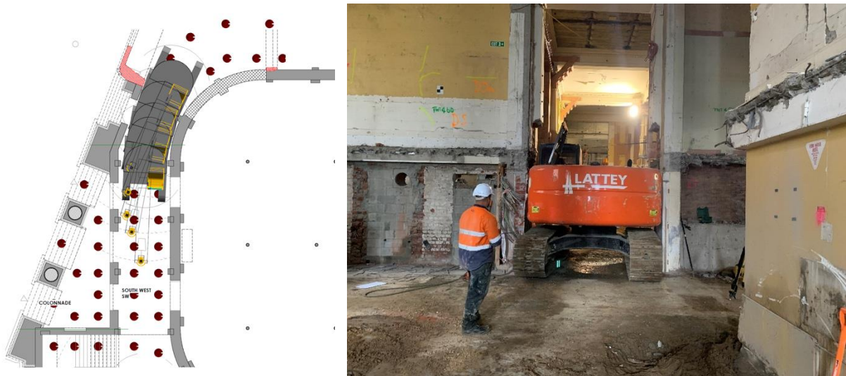
[Figure 7] Modelled route of machinery and reality. There is about 50mm clearance either side of the digger
