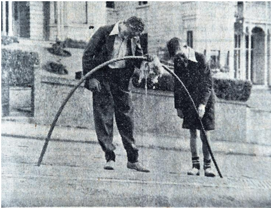
CABLE DAMAGED.—The surge in the cable following this morning's accident to a cable car at the bottom of the High street hill caused the cable to force its way through the centre aperture not far from the Maitland street intersection. The cable was cut and twisted, and will need to be spliced.
