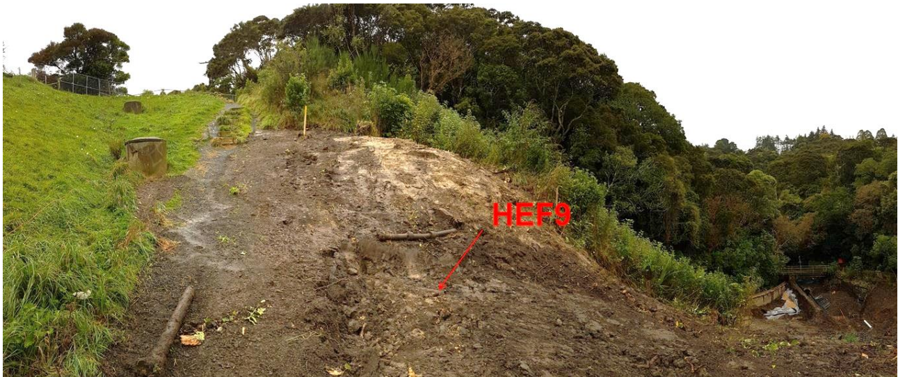
[Figure 5] View of various shallow drainage features exposed during buttress foundation preparation in vicinity of true left abutment, plus shallow collector manholes shown at left of image
