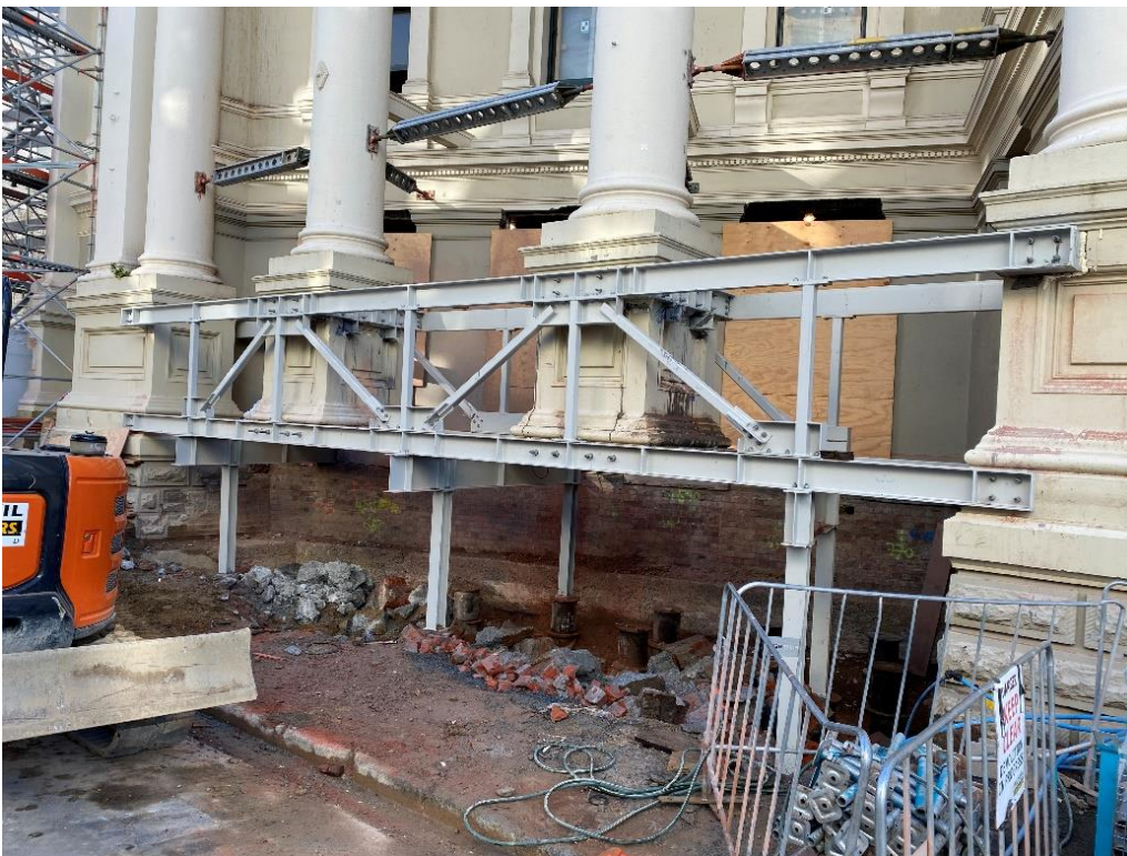
[Figure 20] Colonnade temporary truss in place after demolition of the column foundations
