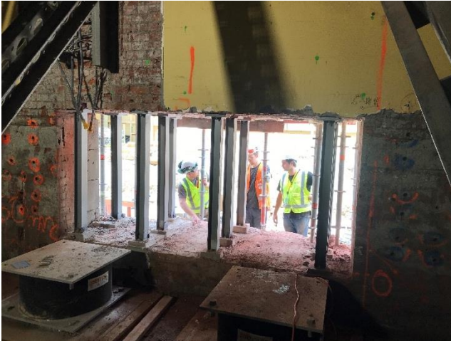
[Figure 16] Temporary works UC props, later cast in with permanent works ground beams
