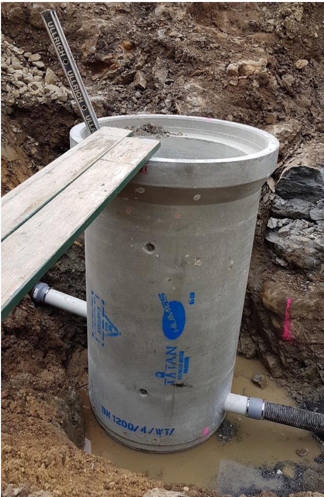
[Figure 7] Addition of western manhole to facilitate monitoring of discovered creek channel drain extending back to dam core trench
