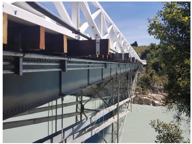
Left: [Figure 8] The original hardwood transoms, showing signs of decay and microbiological growth.
