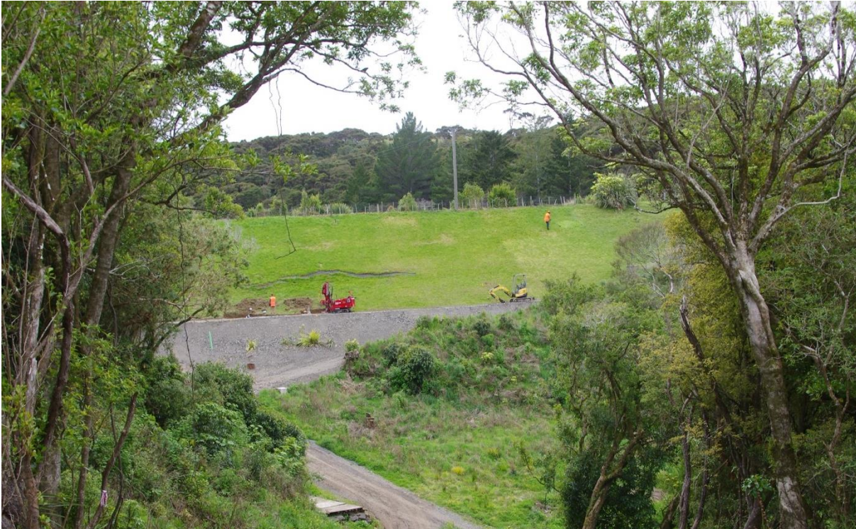
[Figure 3] View of head scarp on embankment shoulder after temporary stabilising fill was placed (investigations in progress)
