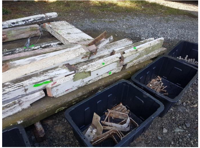
Right: [Figure 22] The balustrade was deconstructed using conservation best practice - each member individually numbered, and its condition assessed for reuse.
