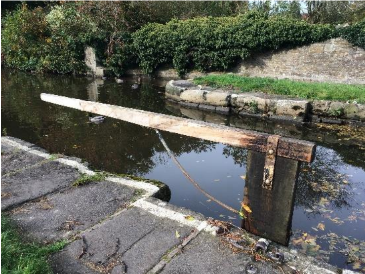
[Figure 12] 'Jack Clough' lock mechanism at Higherland Lock, Leeds and Liverpool Canal
