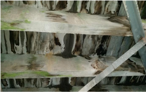
Left: [Figure 27] The original longitudinal decking, viewed from underneath the bridge, showing water damage.
