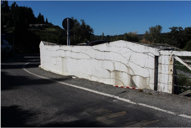
Left: [Figure 12] The damaged parapets prior to repair.
