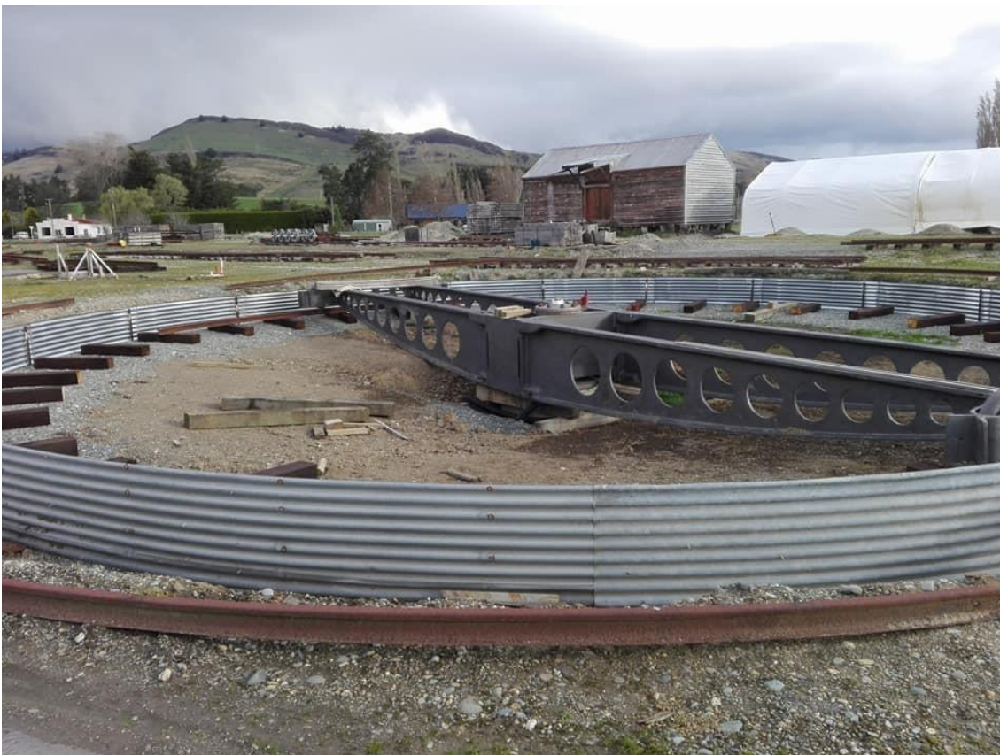
[Figure 14] Sellers turntable No.669 reinstalled at Mandeville but awaiting resources to complete the pit walls and track. Photo by the author.
