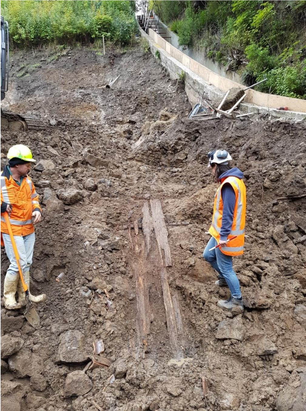
[Figure 4] Exposure of remnants of original 1865 timber flume. (Replacement 1926 concrete spillway in background)
