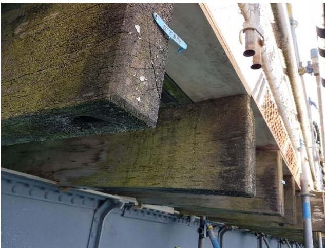
Left: [Figure 8] The original hardwood transoms, showing signs of decay and microbiological growth.
