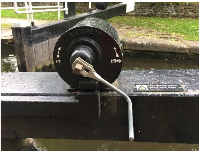
[Figure 11] Windlass and lock mechanism at Salterhebble Guillotine Lock, Calder and Hebble Navigation
