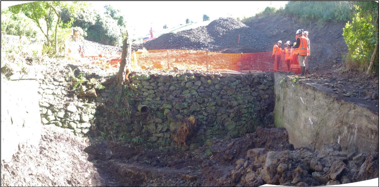
[Figure 2] View looking upstream of the dry-stone wall at the stilling basin portion of the early overflow system following clearing of vegetation, dumped spoil and debris. Current spillway chute is to the right of this image.
