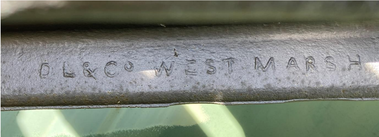
[Figure 21] the Dorman Long brand rolled into some of the angle Irons. Photo by the author.
