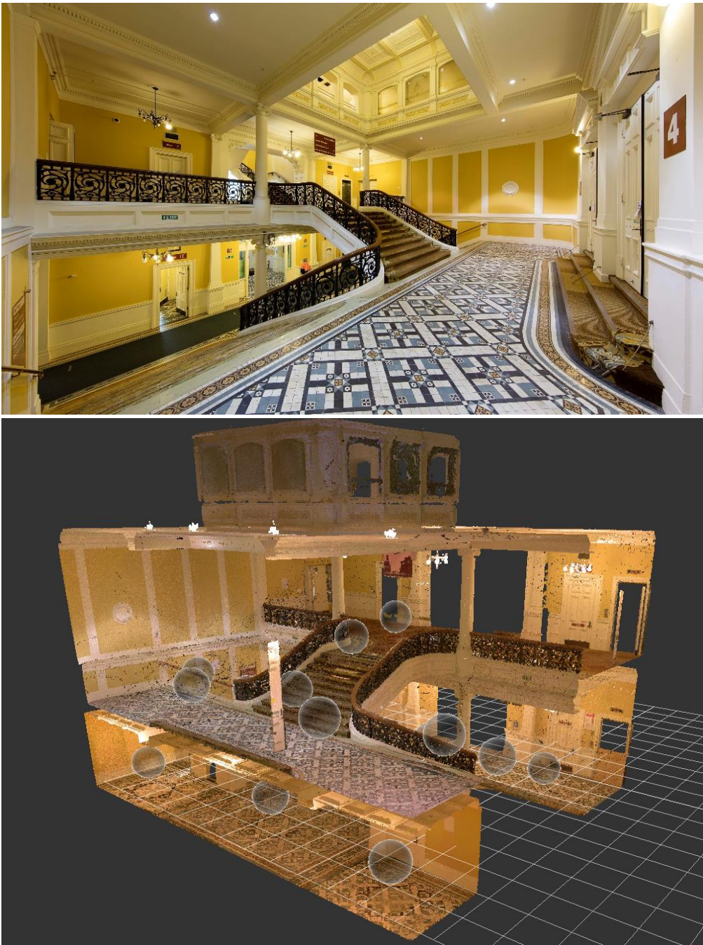
[Figure 13] Photograph and point cloud data of the main stair before demolition. This digital data will be used to make the moulds for rebuilding the stair. Ref also figs 8 and 9
