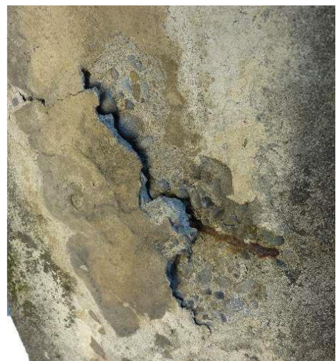
[Figure 40] Mechanical damage to the Opawa Bridge resulting from vehicle scraping and impact.
