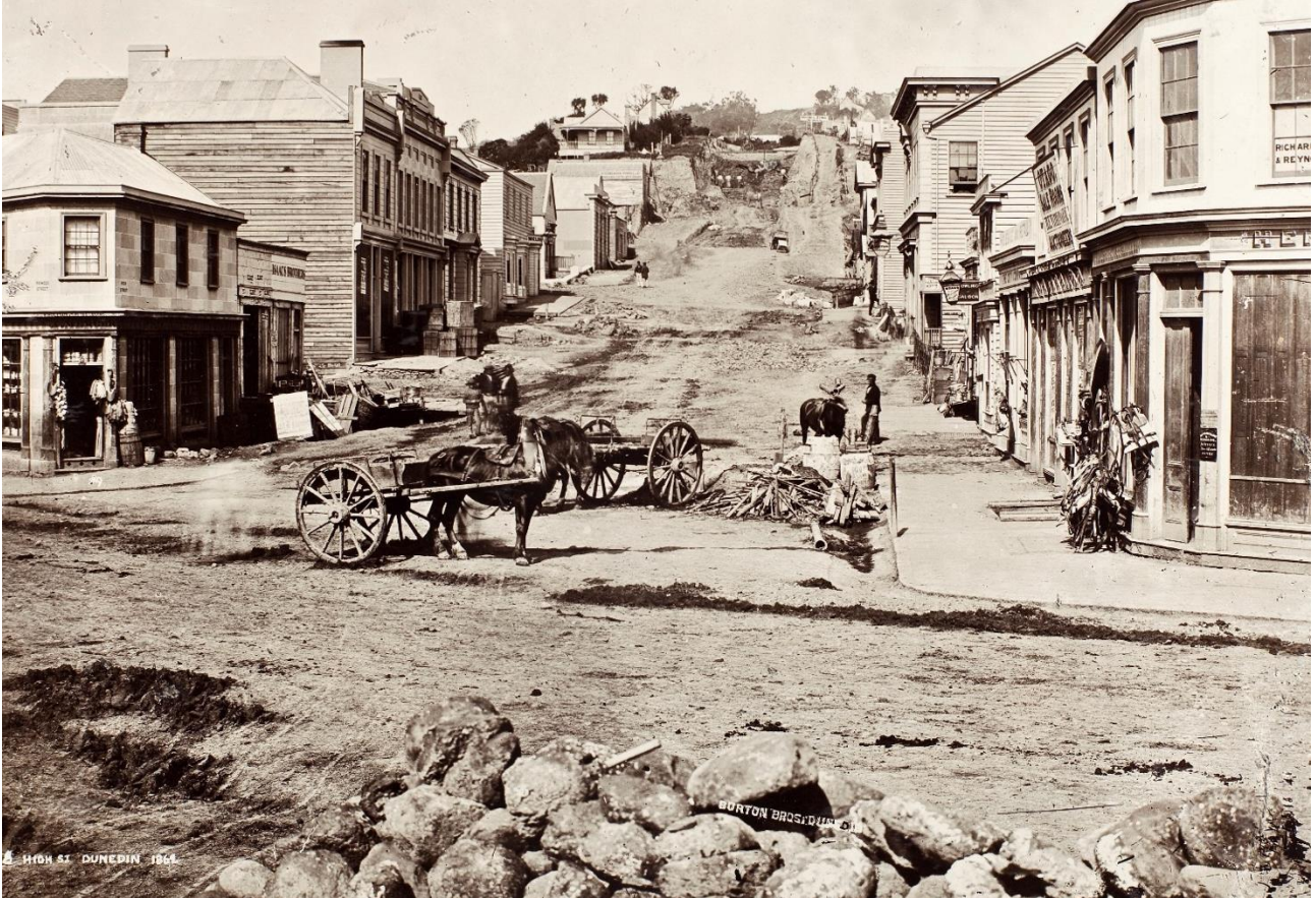
[Figure 7] Looking up High Street from the Exchange (In Princess St.) and part of the Dunedin CBD. A big manual excavation is underway in the middle distance to form High Street. 20 years later, the Mornington Cable Car bottom terminus was positioned just above the upper pair of wheels. High Street, Dunedin, 1862. From the album: Early Dunedin, Meluish - Burton - Muir & Moodie, 1862, Dunedin, by William Meluish, Muir & Moodie studio. Te Papa (O.030520).
