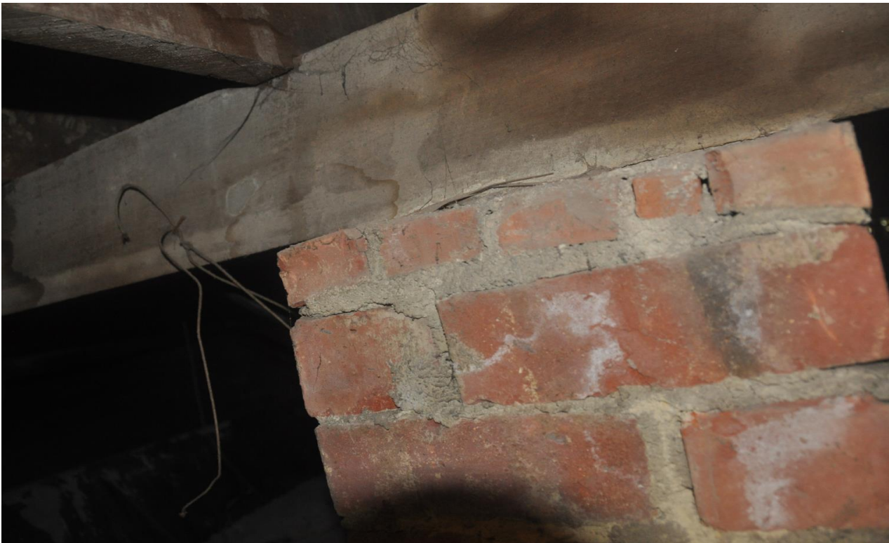
[Figure 8] Photo of existing timber bearer on URM supporting pier. No tie or direct fixing is evident.
