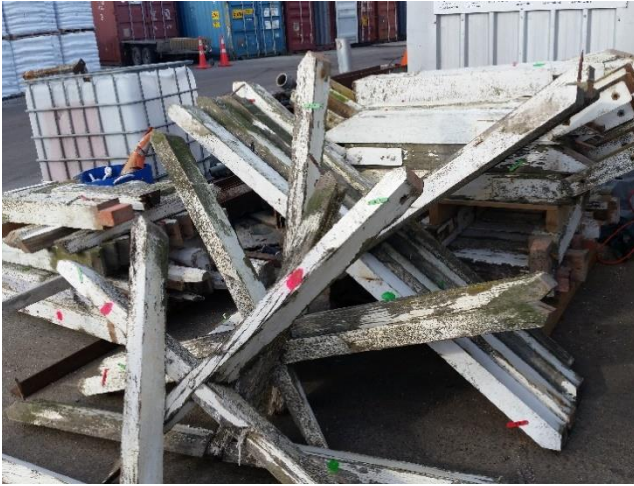
Left: [Figure 21] Removal of the historic balustrades.
