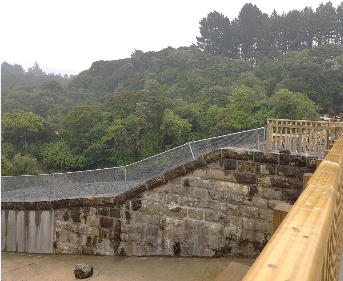
[Figure 11] View of bluestone facing on the raised spillway wall utilising material recovered from site during the project
