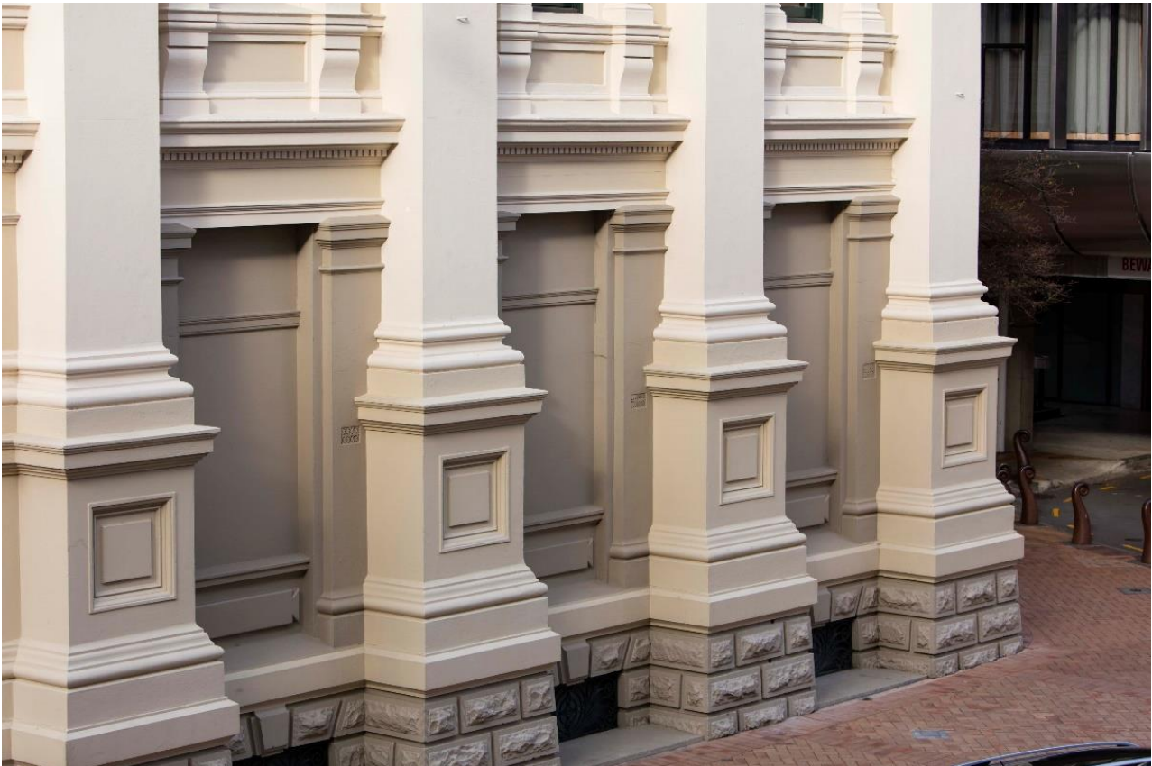
[Figure 14] Exterior of building showing bluestone plinth at base
