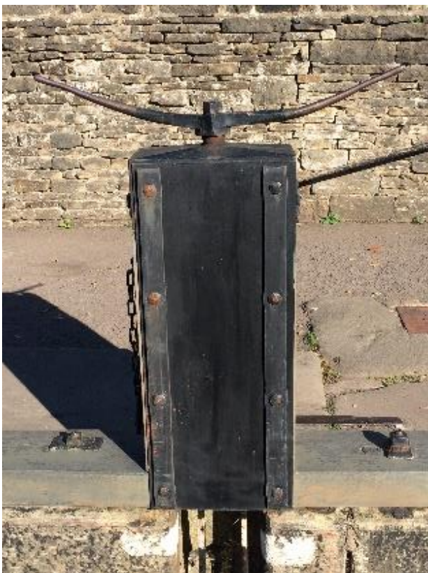
[Figure 14] Box clough lock mechanism, Bingley Five Rise Lock Staircase, Bingley, Leeds and Liverpool Canal
