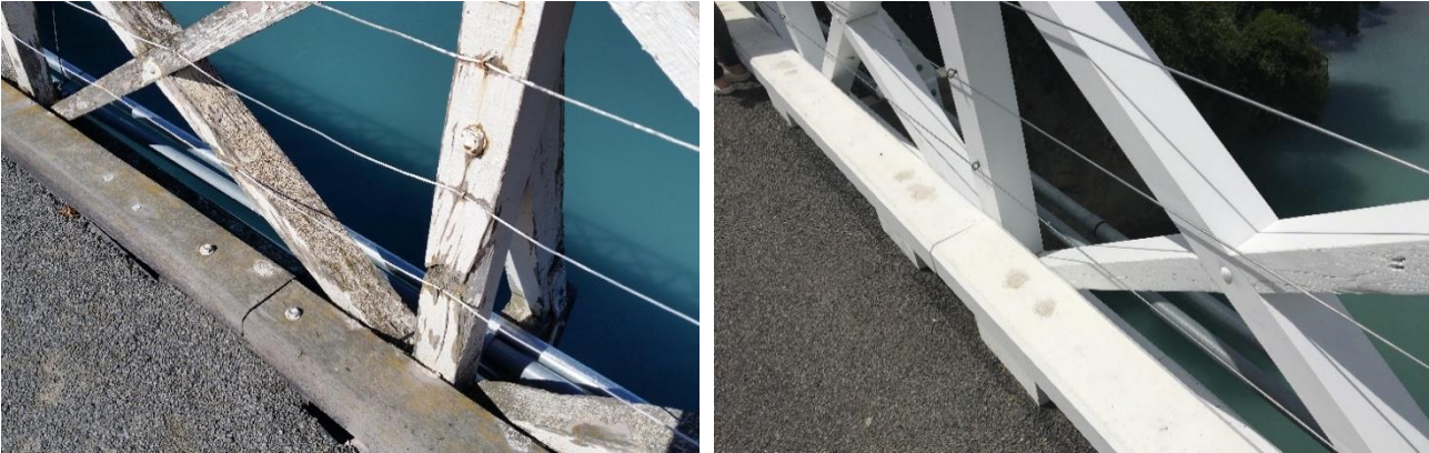
Left: [Figure 19] The damaged balustrade and timber kerbing prior to repair. Right: [Figure 20] The repaired balustrade, with timber kerbing.
