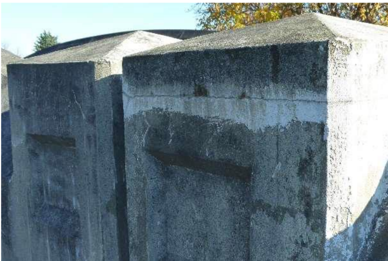
Left: [Figure 41] Typical example of cracking on the Opawa Bridge prior to restoration works.
