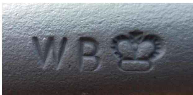
[Figure 22 and 17] Two variations of a works stamp on a joint plate and on a tie-rod. Photo by the author.
