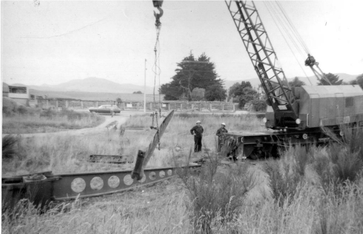
[Figure 8] Dismantling a turntable. A comparatively modern photo, thought to have been taken at Tuatapere in 1977 with the turntable destined for Clyde. While this is a larger 55ft table manufactured in New Zealand, it retained the modular construction exactly as designed by William Sellers. From the author's own collection.
