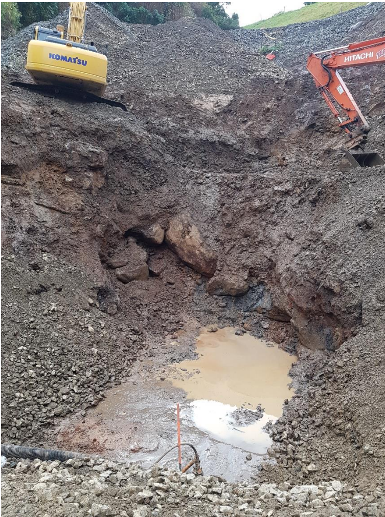
[Figure 6] Buttress foundation preparation at creek channel showing basalt boulders
