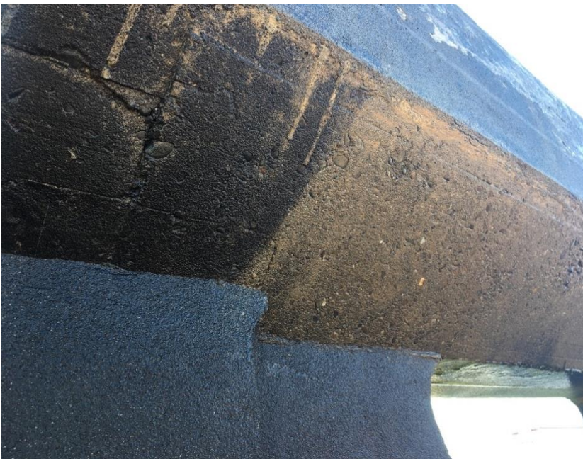
Left: [Figure 46] Cleaning the Opawa Bridge with the Thermatech system.
