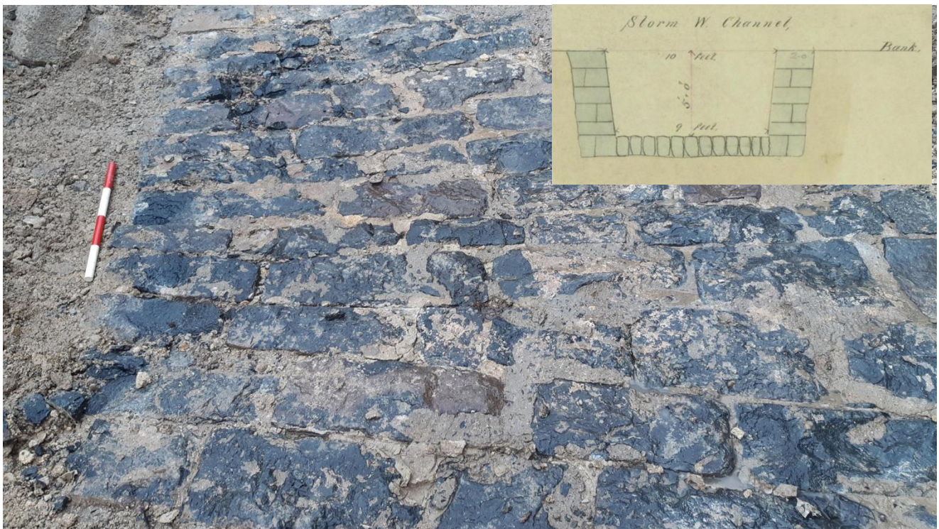
[Figure 8] Bluestone pitching exposed under later lining
