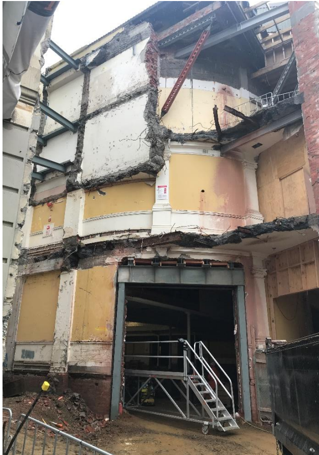
[Figure 15] Openings in URM wall for access and equipment needed inside
