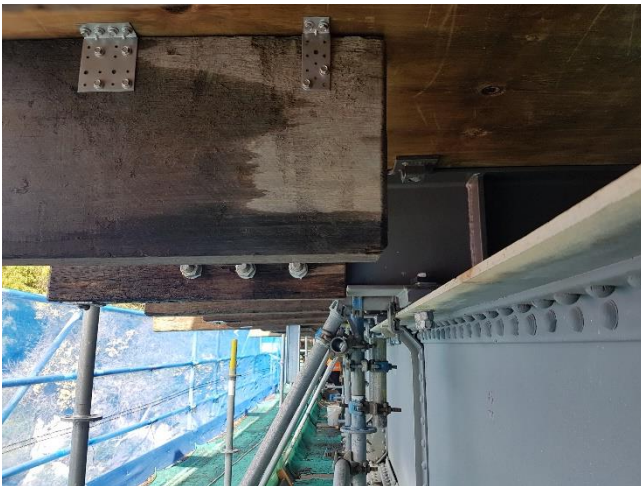
Left: [Figure 10] Transoms without steel substructure attached to the deck to retain the aesthetic features of the bridge.
