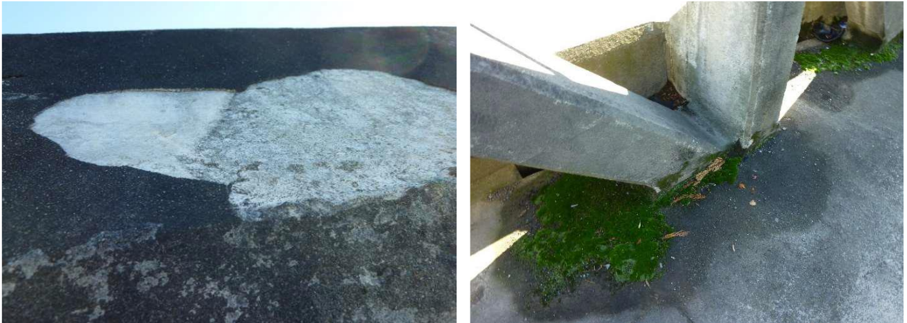
Left: [Figure 43] Delamination of surface render on Opawa Bridge prior to restoration.
