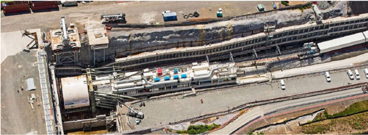
[Figure 15] 87m long Alice tunnel boring machine ready to start its journey in December 2013. NZTA picture.
