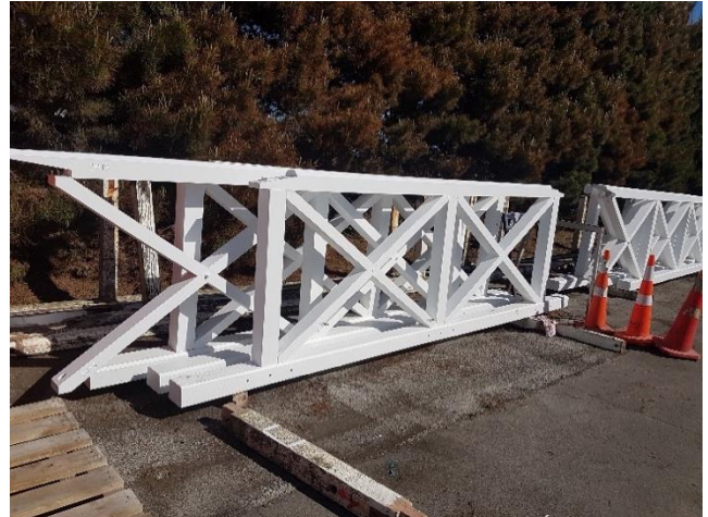
Left: [Figure 23] Reconstruction of balustrades, incorporating historic fabric where possible.
