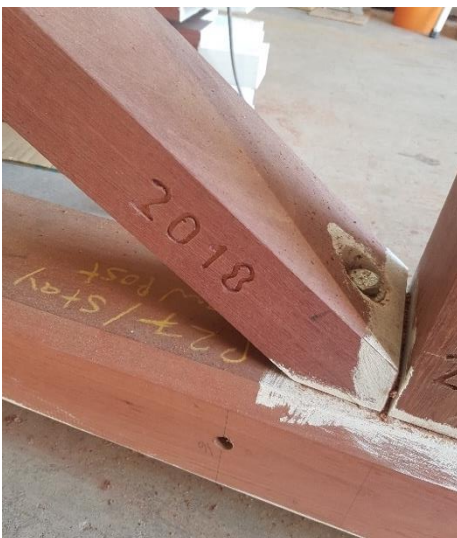
Left: [Figure 25] Date stamping of the new balustrade.
