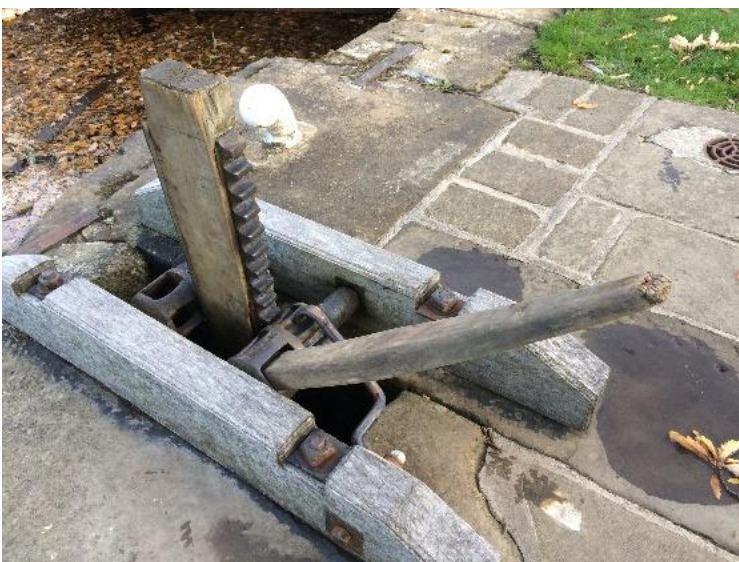
[Figure 13] Handspike and lock mechanism at Kirklees Low Lock, Calder and Hebble Navigation
