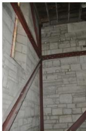
[Figure 10] Reinforced concrete internal skin strengthening of tower, with photos of the existing seismic steel bracing to be replaced.
