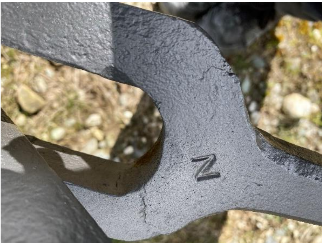
[Figure 20] Possibly an Inspectors mark, only found on a few of these forked rod ends. Photo by the author.
