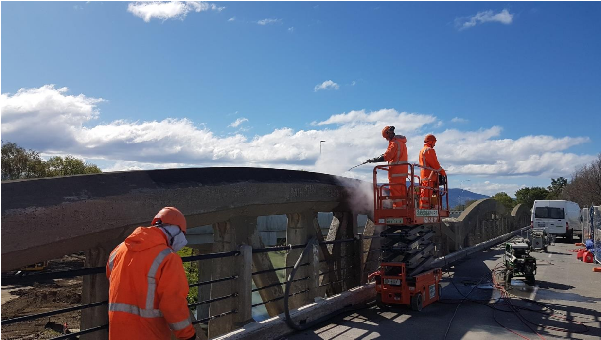
[Figure 45] Cleaning the Opawa Bridge with the Thermatech system.
