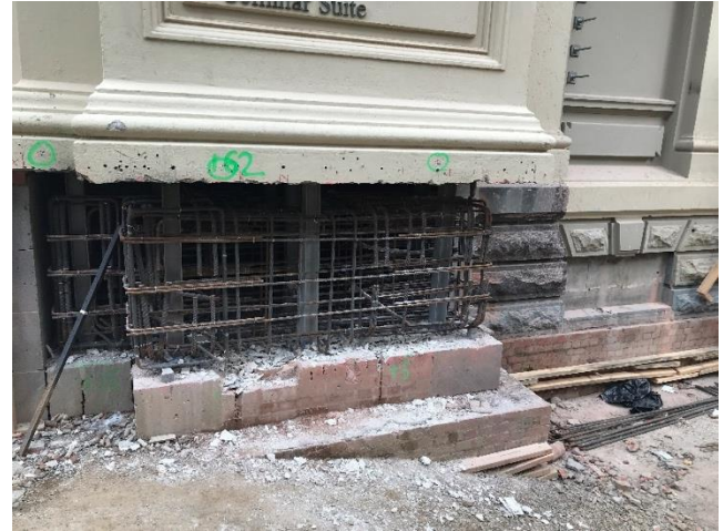
[Figure 16] Temporary works UC props, later cast in with permanent works ground beams
