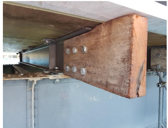
Left: [Figure 10] Transoms without steel substructure attached to the deck to retain the aesthetic features of the bridge.
