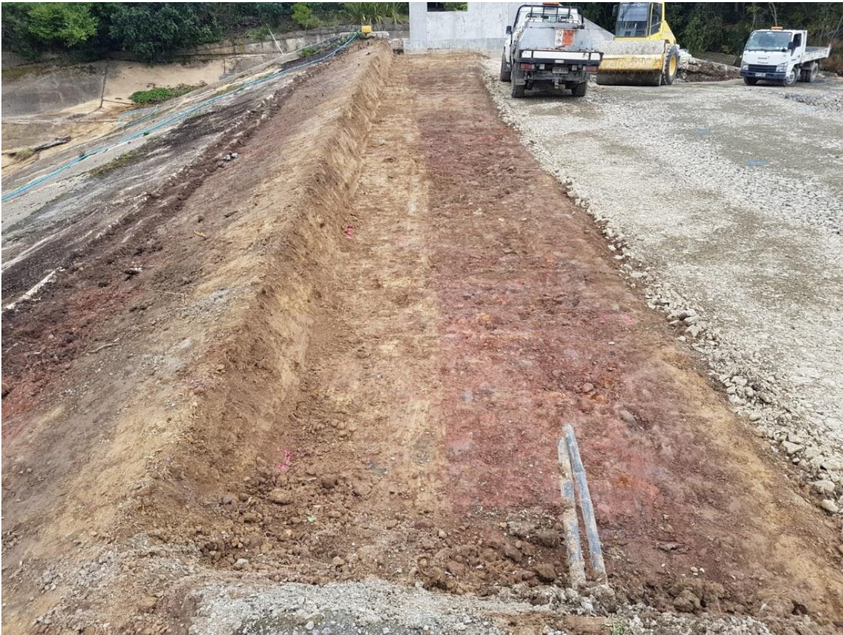
[Figure 9] Stripped dam crest exposing trenched core capping zone. Buttress placement to right of image has temporary cover extended over obscured new sand and gravel filter layers below
