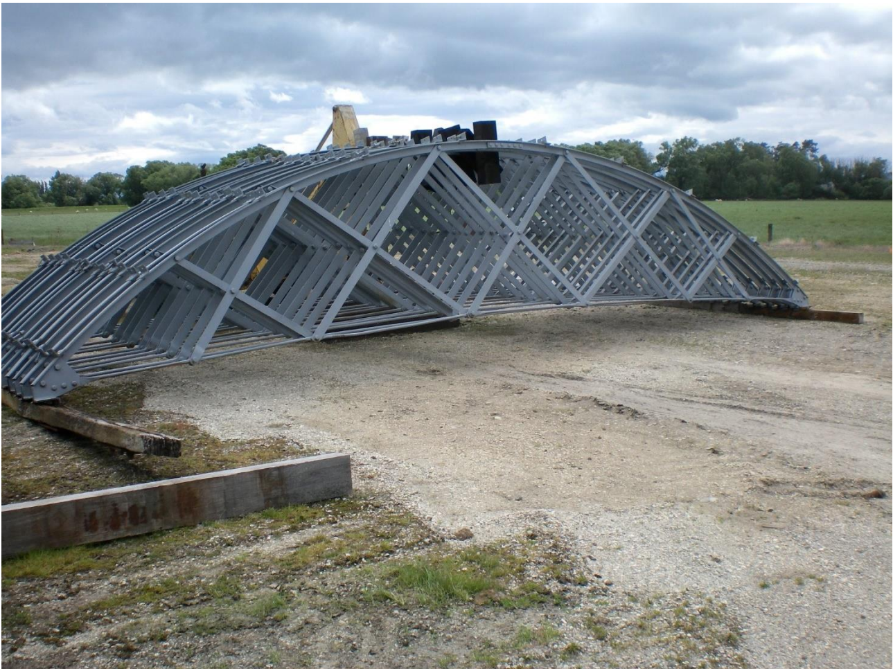
[Figure 15] The first set of trusses after cleaning and painting, ready for erection. Photo by the author.
