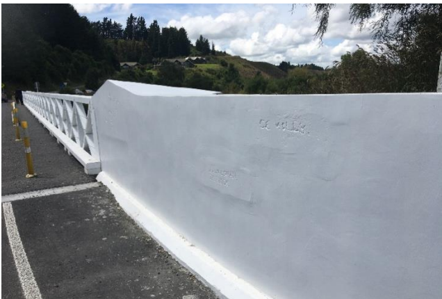
Left: [Figure 14] The repaired parapets, repainted white to improve visibility.
