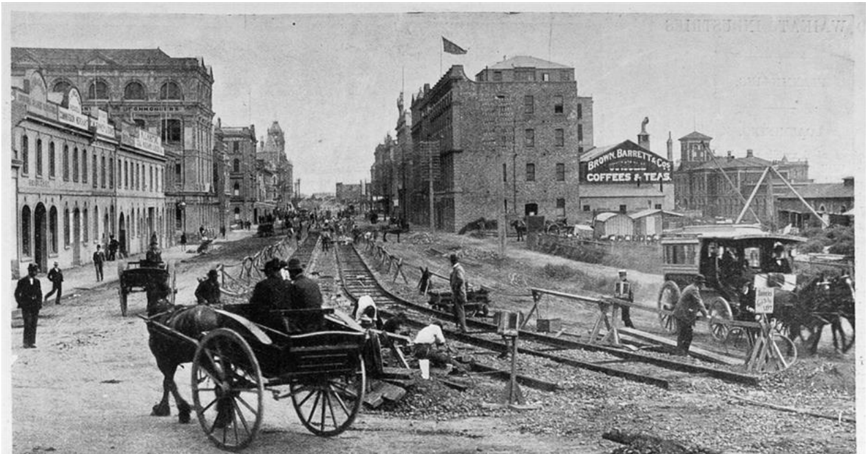
[Figure 4] Laying tram tracks in Custom Street Auckland November 1901. Sir George Grey Special Collections AWNS-19011107-5-1
