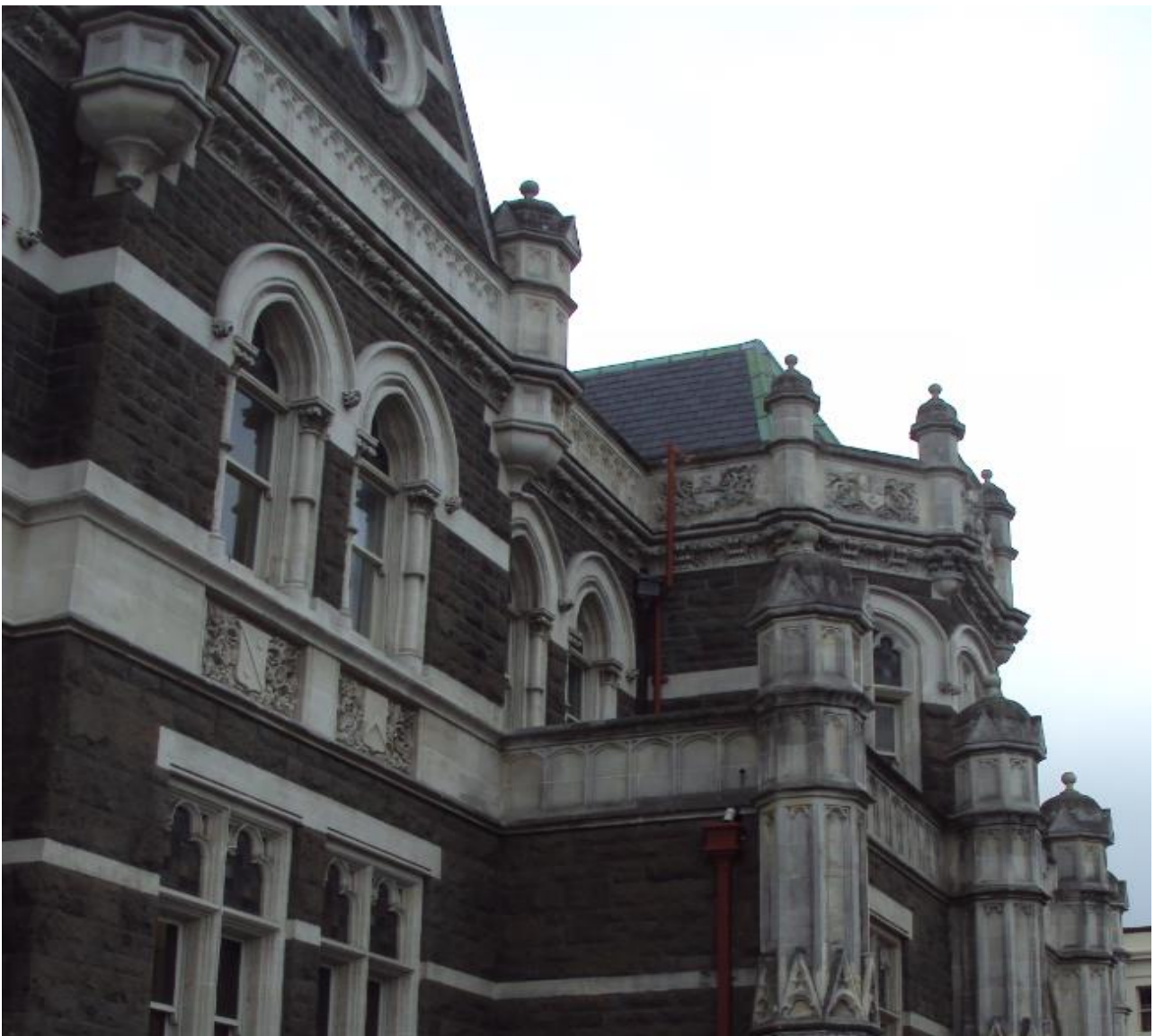
[Figure 11] Photo showing typical URM and Oamaru stone parapets and ornaments which required additional seismic restraint.
