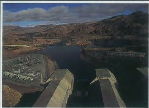
Benmore Power Station (DC switchyard on right of picture in background)
