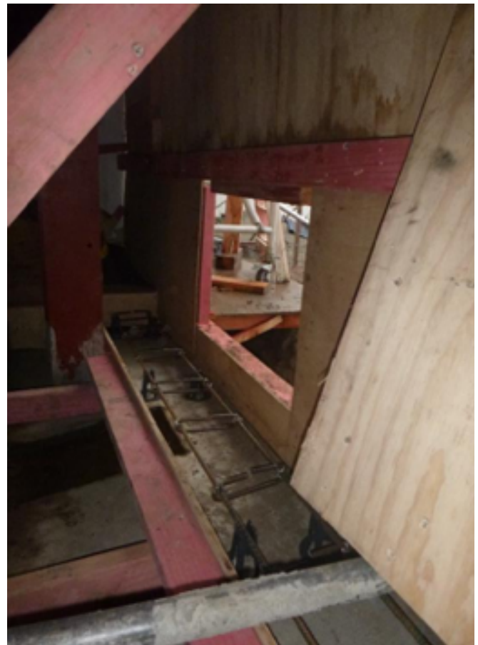
Photo 4 Nib wall cage and reinforcing
