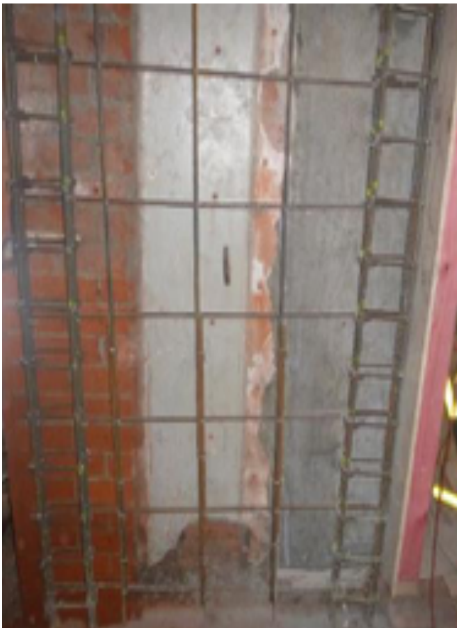
Photo 3 Showing holes for hooks to be inserted
