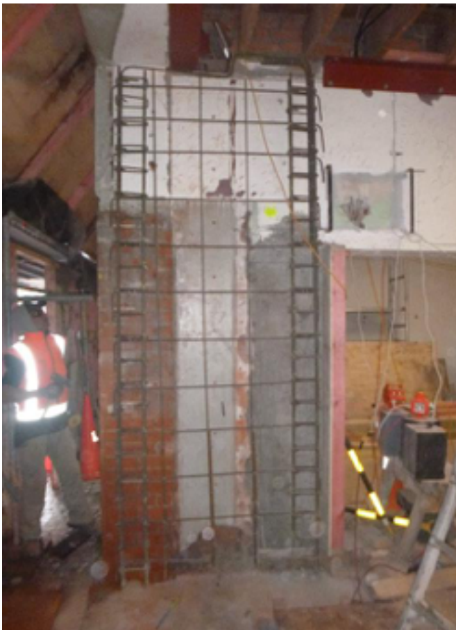
Photo 1: Overview of wall to be sprayed
