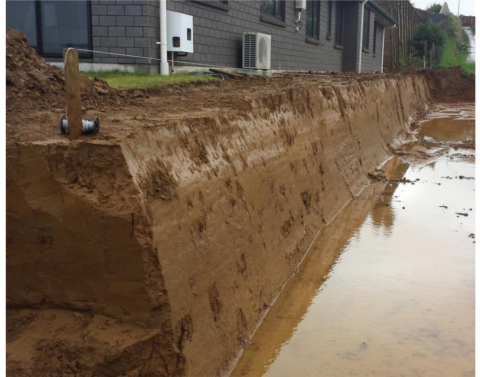
Figure 3: Image taken February 2019 – note remedial fill at the toe
