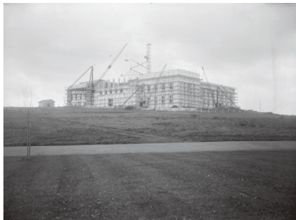
View showing the north and west faces of the Auckland War Memorial Museum under construction, 1927.
