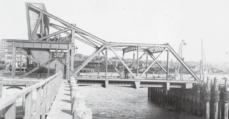
Rolling lift bridge viaduct to Freemans Bay with the bridge closed, 29 June 1932. Auckland Harbour Board collection, NZ National Maritime Museum
