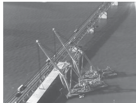
Auckland Harbour Bridge attachment of bridge extension, 1967. Courtesy of Geosmart Ltd, Auckland
