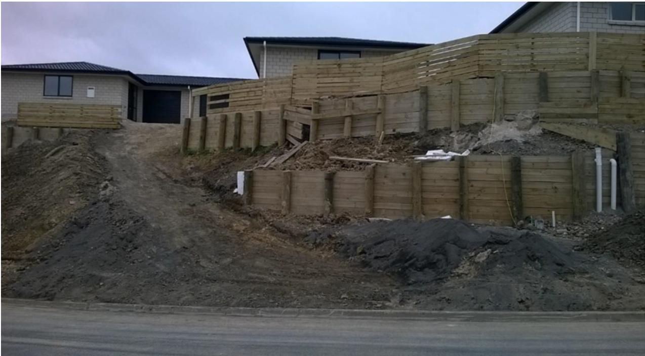
102. In response, Mr Cameron said the collapse was due to excavations in front of the wall, not due to his design or sign-off. In his submissions to the Disciplinary Committee, he said a drainlayer excavated the backfill behind the retaining wall and backfilled it with poor quality backfill after he had inspected and certified the wall.
